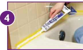
4 Apply caulk. Smooth bead to desired finish.
