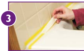
3 Once aligned, pull off the white release liner at a 75-degree angle, exposing the yellow tape. The area not covered by the yellow tape forms a perfect gap over the joint to be caulked.
