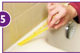
5 Immediately peel off yellow tape and dispose of it.
