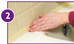
2 Apply tape yellow side down to the tub surface, flush with the adjoining wall.
